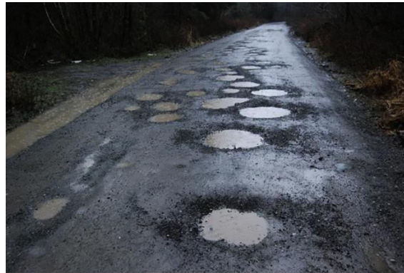
Fig. 1: Road Pothole
