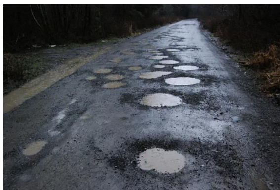
Fig. 1: Road Pothole
